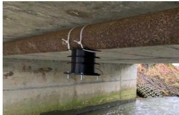
**Figure 3: One of our water level measurement stations installed beneath a bridge in a flood-prone area.**
