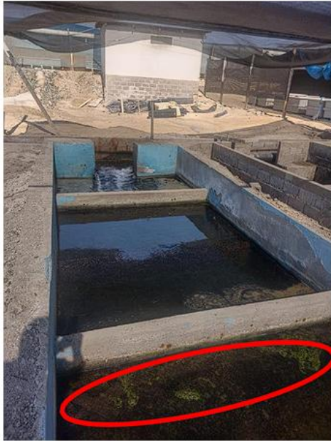
Image 6: Decanting tank at the beginning of the experiment (presence of particulate organic matter and dissolved organic matter).
