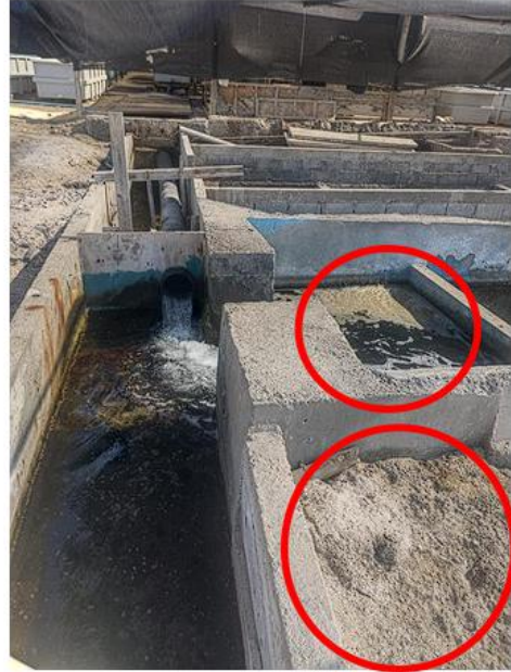
Image 6: Decanting tank at the beginning of the experiment (presence of particulate organic matter and dissolved organic matter).
